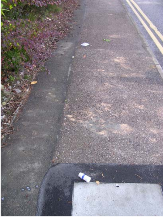
Lochavullin Road continued
